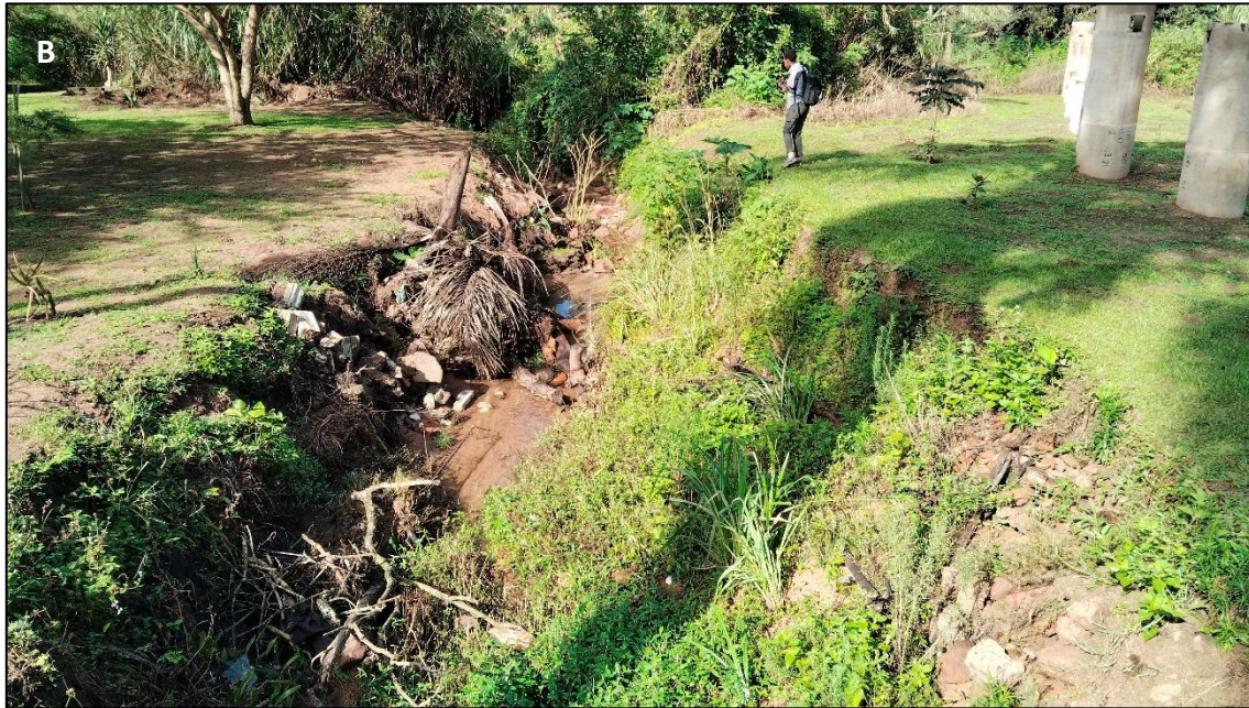
Figure 7-3 A) Evidence of attempts to stabilise bank erosion along Riparian Channel 2. B) Extensive channel incision at the toe of Riparian Channel 2.
